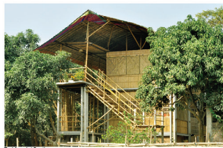
End facade South
