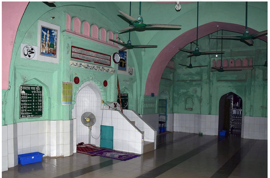
Figure 05: Interior condition of the mosque / Photography Year: 2015.
