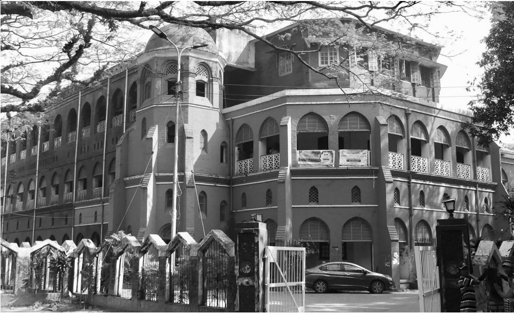
Fig 2: The view of CRB from the main gate.
