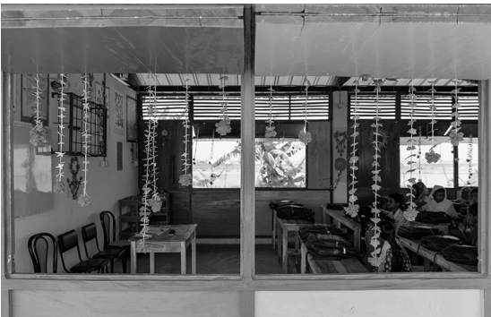
THE COOLING WINDOWS CAN EASILY BE SHUT DURING CYCLONES
