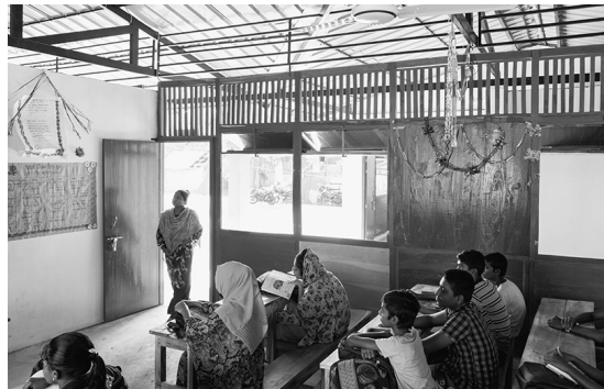
CLASSROOM TOPPED BY STEEL ROOFING
